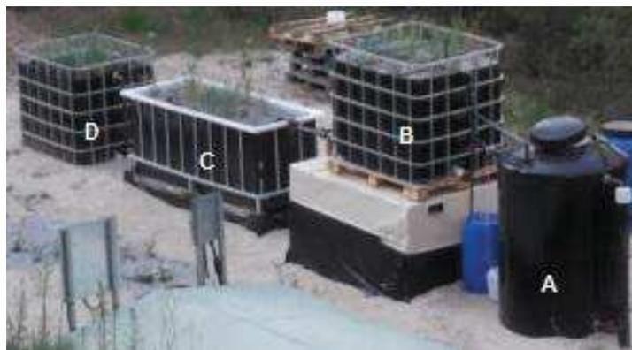
**Figure 1.15.** Hybrid constructed wetland. A) Influent mixer; B) vertical subsurface flow CW; C) horizontal subsurface flow CW; D) surface flow CW.
