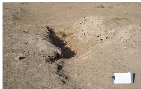
Earthworks at Grid B
