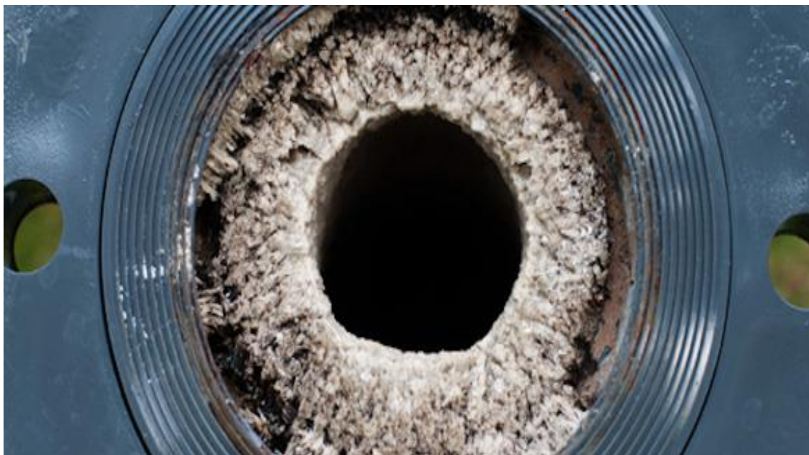
Figure 2. Wastewater Treatment Struvite Plugged pipeline. (CED)
