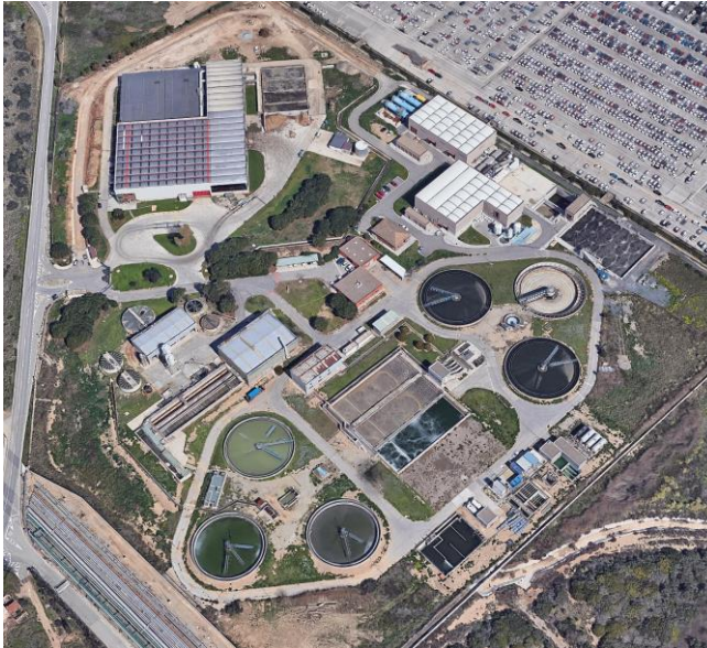
Figure 15. Aerial view of Vilaseca/Salou EDAR (Google Earth, 2020. November 2020)
