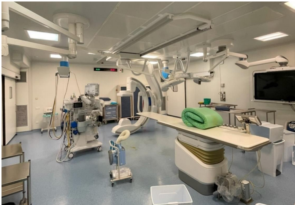
Figure 13 Studied Operating Room from Hospital Germans Trias i Pujol
