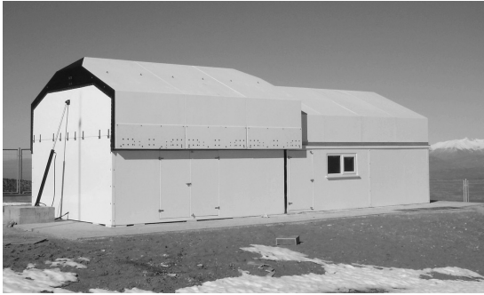
Figure 3. Reinforced glass-fiber enclosure at OAdM.
