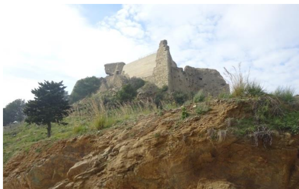
Figure 4: The fort after the reconstruction carried out between 2002 and 2010 (Arxiu Didpatri-UB).
