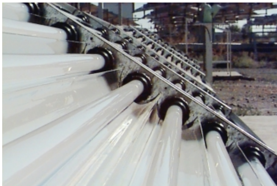
Figure 4.10. Detail of a collector CPC where the configuration of the tubes reactors is observed
