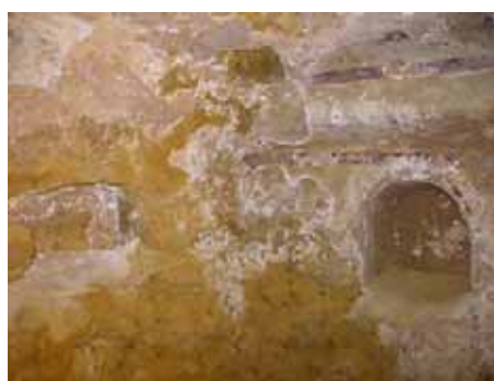
Figure 3. Tomb of Postumio. Note the deterioration of mural paintings and the
