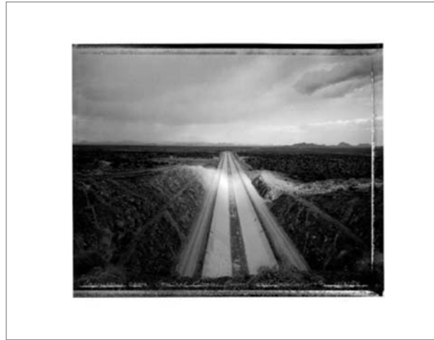
Fig.124 Engineering oasis, Central Arizona Project canal awaiting water, 10/21/84
