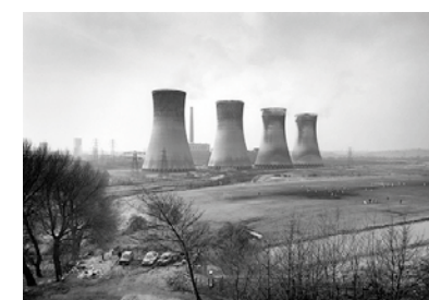
Fig.261 Agecroft Power Station, Salford, 1983
