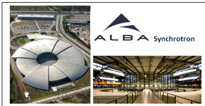
FIG.4. ALBA Synchrotron is a peculiar building with 270 m of circular perimeter located in Campus of Universitat Autònoma de Barcelona. (ALBA intranet, material available for students)
