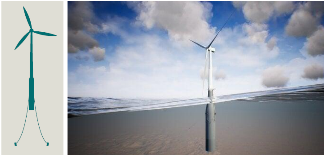
Image 2: Spar buoy figure (IRENA 93 ) and Hywind Tampen's computer-animated floating spar wind turbine (Aker Solutions 94 ).
