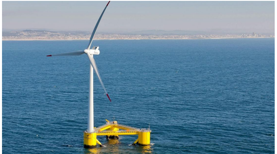
Image 4: Semi-submersible figure (IRENA 97 ) and Principle Power's WindFloat semi-submersible wind turbine (Principle Power 98 ).
