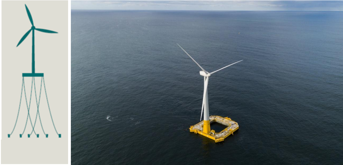
Image 3: Barge figure (IRENA 95 ) and BW Ideol's Floatgen barge wind turbine (BW Ideol 96 ).
