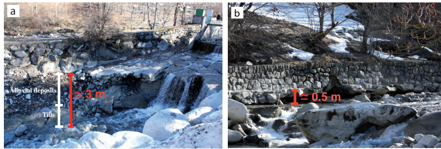
Figure 8. Erosion evidence in the Valarties River (photos Glòria Furdada, January 2014). (a) The 3.5 m incision downstream of the gauging station (partly related to local turbulence) allows the outcrop of fluvial and glacial deposits. (b) The incision is about 0.5 m below the channelization dyke upstream of the gauging station.
