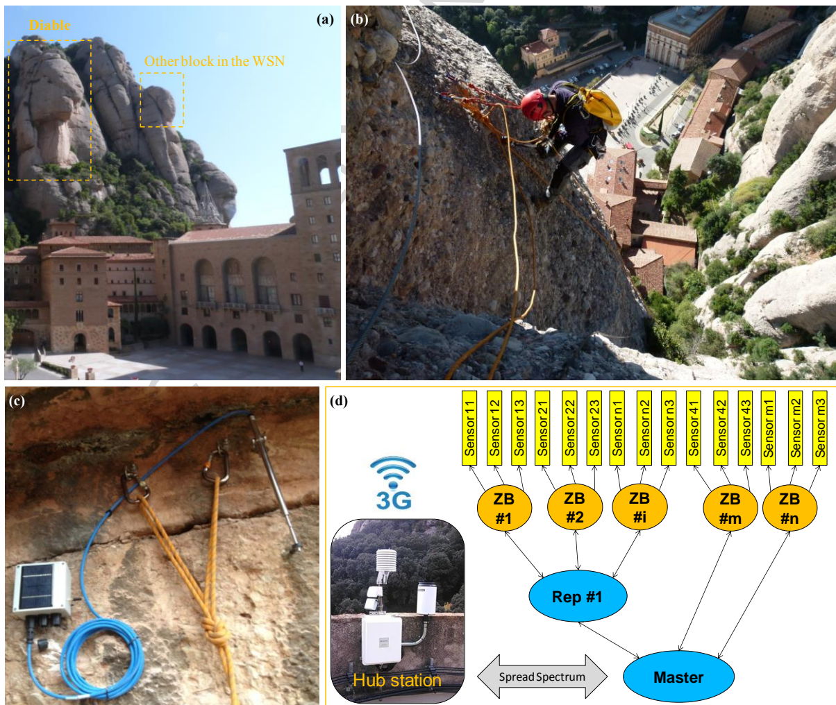
Figure 6. Location of the Diable blocks above the monastery (a). Monitoring of the block's joints with crackmeters, bar-tiltmeters and wire-extensometers installed using rope access works (b). Configured network based on ZBLoggers connected to sensors (c) and wireless communication through repeaters and a master to the hub station connected to Internet by a 3G mobile communications system (d).
