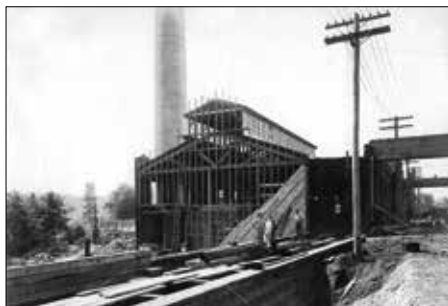
D. Electrical plant, next to the train tracks.
