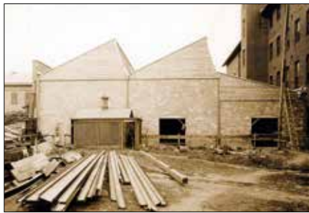
B. Annex to the central buildings.
