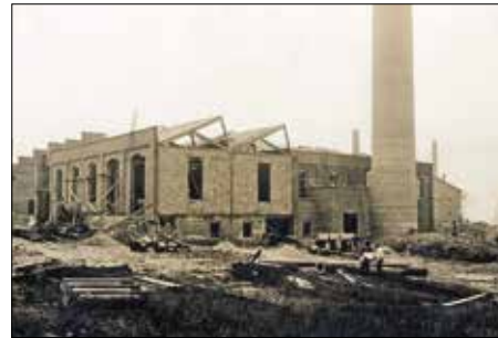
C. Electrical plant premises.
