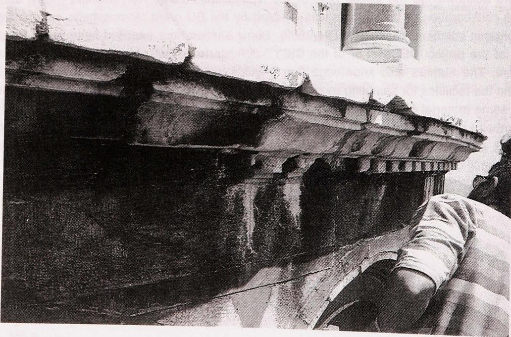
Fig. 2: Dark patina under a cornice. The zones under the joints of the elements of the cornice have been washed because the decay of the joint mortars concentrates the running water.
