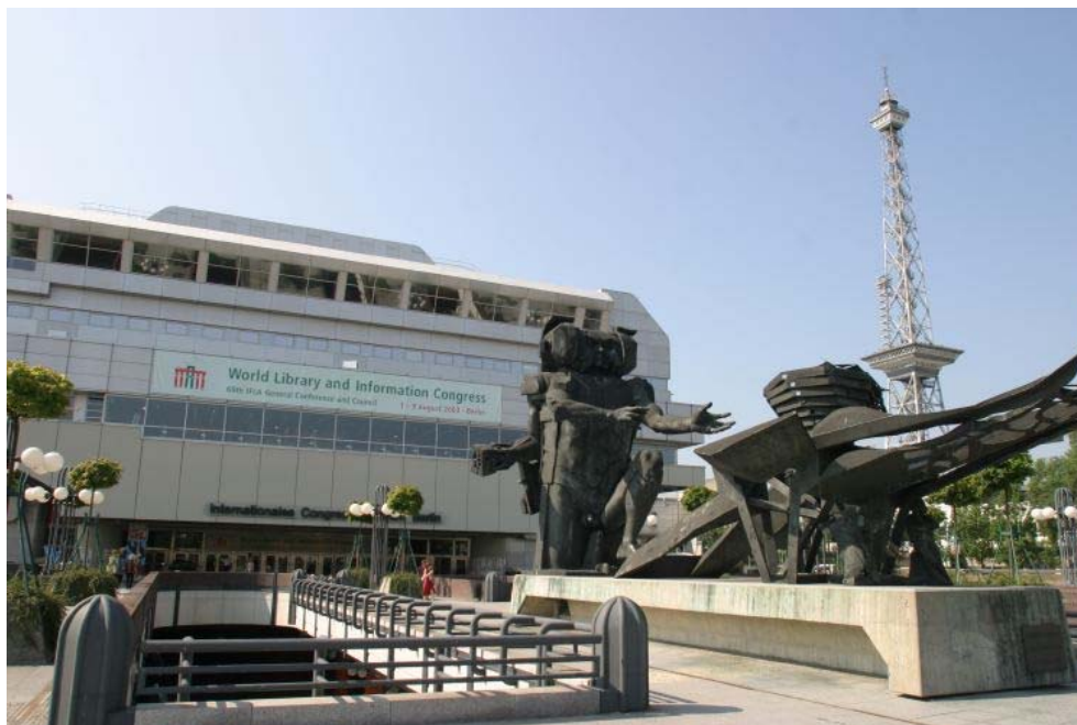
Figura 1. Vista general de l'International Congress Centre (ICC). (c) BDB-IFLA 2003/Dirk Deckbar
