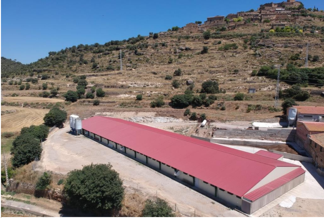
Figure 7. South-vision of the roof where modules will be developed.
