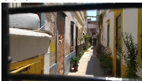
Figure 3 - Common area of property to be demolished at Carrer Ramon Turró
