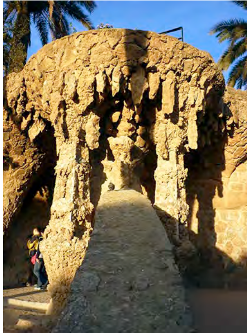
Fig. 1. The set at the end of the Laundry Room Portico, seen from where the Hypostyle Room is located.
