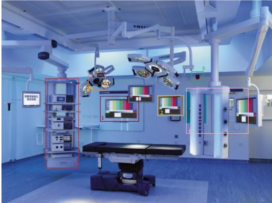
Figure 8. Audiovisual integration of an operating room powered by Olympus. Several components can be identified: 1. Wall monitor; 2. Medical-grade monitor; 3. Ambient camera (PTZ); 4. Lamp camera; 5. Audiovisual column; and 6. Operating Room Technical Panel. Source: 40.
