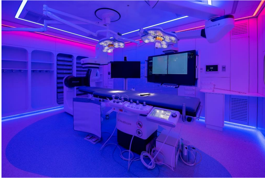
Figure 7. Hemodynamics Operating Room where two Operating Lights, a Laminar Light, and a Perimeter Light, both ceiling and floor, can be clearly observed. Own source.
