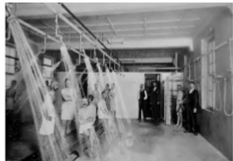
Figure 2: Bathroom of the Utica Psychiatric Centre (Image: The Rain-Bath William Paul Gerard, 1895).
