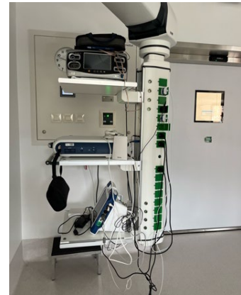
Figure 12: Ceiling-mounted storage system with power outlets.
