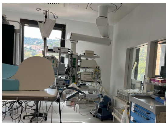
Figure 27: Ceiling-mounted storage system from Hospital Universitari Vall d'Hebron.
