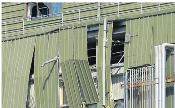
Figure 13: The north side of Production Building No. 2 (PB2) after the incident. Source: Runaway chemical reaction at Corden Pharmachem, Cork
