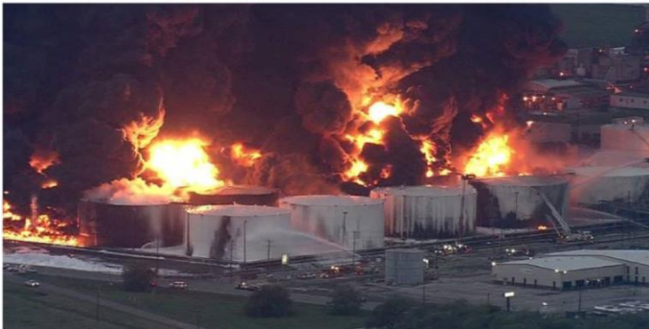
Figure 7: Fire and domino effect caused by the butane leak. Source: LCC ACCIDENT
