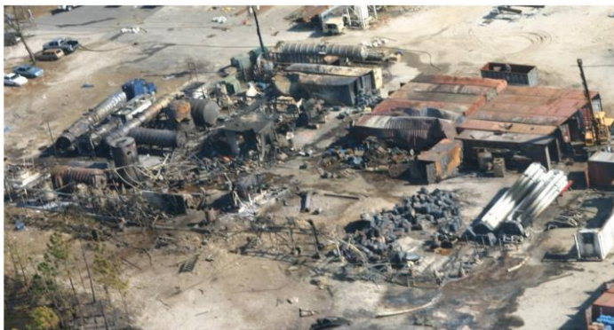
Figure 15: Chemical plant of T2 Laboratories after the accident caused by the uncontrolled reaction on December 20, 2007. Source: T2 Laboratories Inc. Reactive Chemical Explosion
