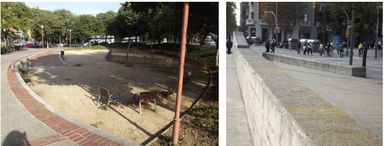
Fig.50 Plaça Pablo Neruda view of the playground (left). The sculpture-like concrete wall at the vertex of the square (right).
