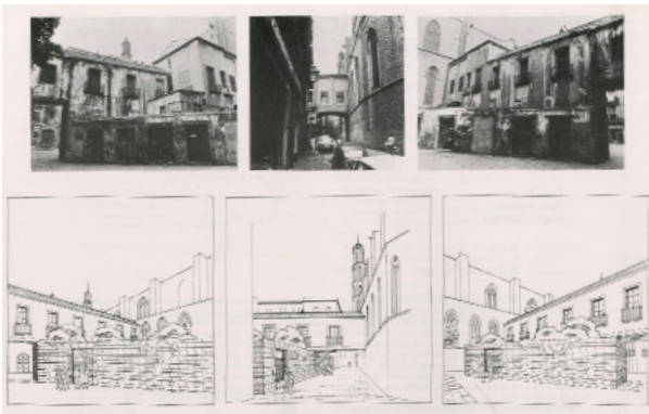
Fig.43 The square before the demolitions.
