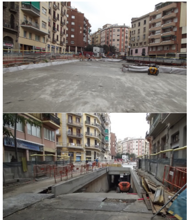
Fig.52 Plaça de Navas is under total reconstruction (2011)
