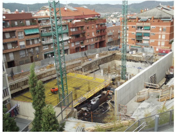
Fig.79 Construction of the subterranean parking in the lower level
