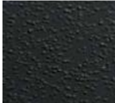
Figure 3.4. Paint defect. Solvent popping. (Image from Paints defects , reference 4)
