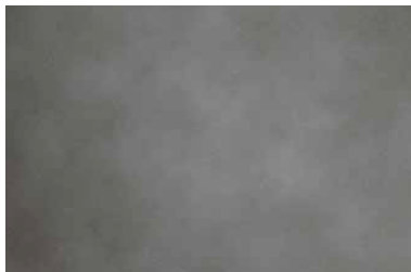
Figure 3.3. Paint defect. Clouding. (Image from Paints defects , reference 4)
