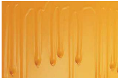
Figure 3.2. Paint defects. Sagging. (Image from Paints defects , reference 4)
