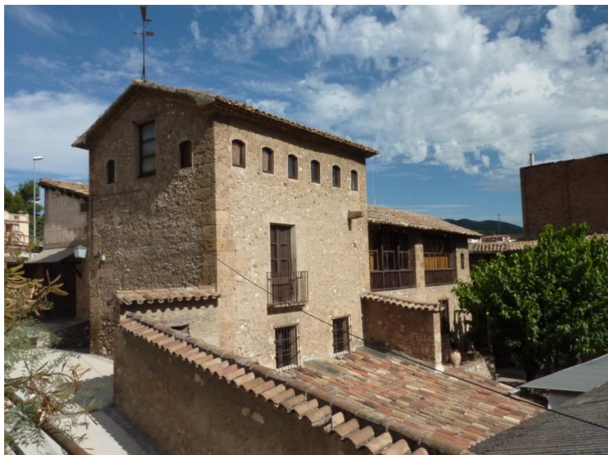
Vista frontal: edifici paperer i galeries (2013)
