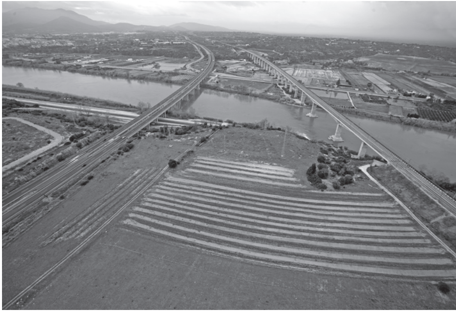
Fig. 6 Aerial photograph of the La Palma site (2007) next to the River Ebro, now crossed by the freeway and railroad. The parallel lines in the foreground are due to the systematic stripping of layers.
